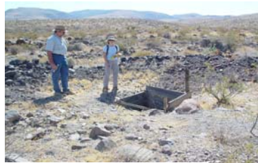
Dug well requiring rehabilitation
