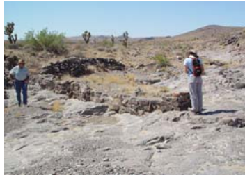
Rock and mortar dam requiring rehabilitation
